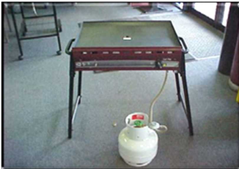
Figure 10: An example of an unsuitable appliance installation.
